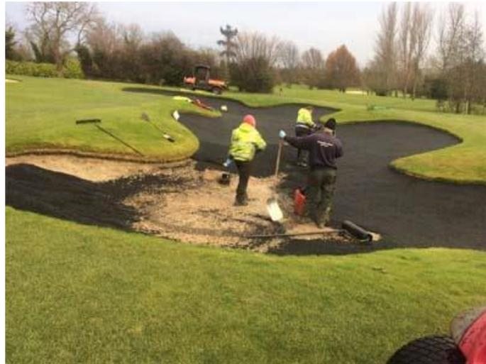
As part of our ongoing bunker improvements we carried out further membrane installations on the 2<sup>nd</sup>, 3<sup>rd</sup>, 4<sup>th</sup> and 5<sup>th</sup> greenside bunkers. This has proved to be a very successful bunker lining technique in delivering consistent quality of bunker playability in all-weather events.
