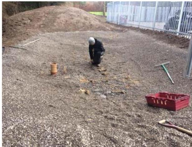
As part of our secure compound project we built a wash down cleaning area for the machinery and sprayer. The waste water from this work is fed into a reed bed pond that is constructed using Norfolk reeds (*Phragmites Australis*). These plants filter the contaminated water as it passes through its root mass with the result that clean water reenters the aquafier.
