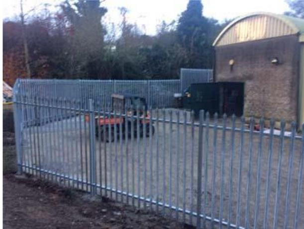
In order to better secure our machinery workshop and yard we created an expanded concreted compound surrounded by 2.4m high security fencing. As part of this project we levelled and resurfaced the avenue up to the workshop
